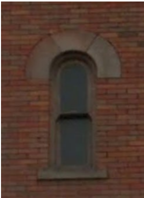
Third-floor accent arches
